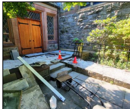
Refurbishing of Chapel Entry Walkway
