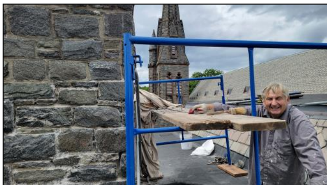
Eddie, the mason, working on chimney to fireplace in Jason's office.
